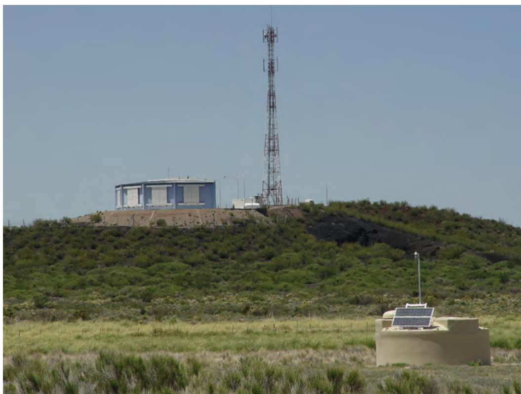
FIGURE 8.10 Pierre Auger Observatory of ultrahigh-energy cosmic rays in Mendoza Province, Argentina. Shown is one of the particle detector tanks of the 1,660 units covering 3,000 square kilometers and one of the four fluorescence telescopes that overlook the array. SOURCE: Courtesy of the Pierre Auger Observatory.
